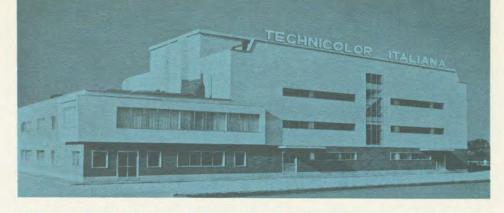
COLOR FILM PROCESSING PLANT, ROME, ITALY, is located on the outskirts of Rome, covers a floor area of 49,000 sq. ft. and has complete facilities for the manufacture of 72 million feet of release prints per year by the dye transfer process. All aspects of layout and construction of the buildings were under the control of the Engineering Department, and all items of processing equipment were both designed and constructed by that group.
